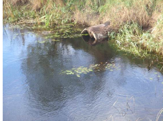
Culvert discharge to Mongagh River
